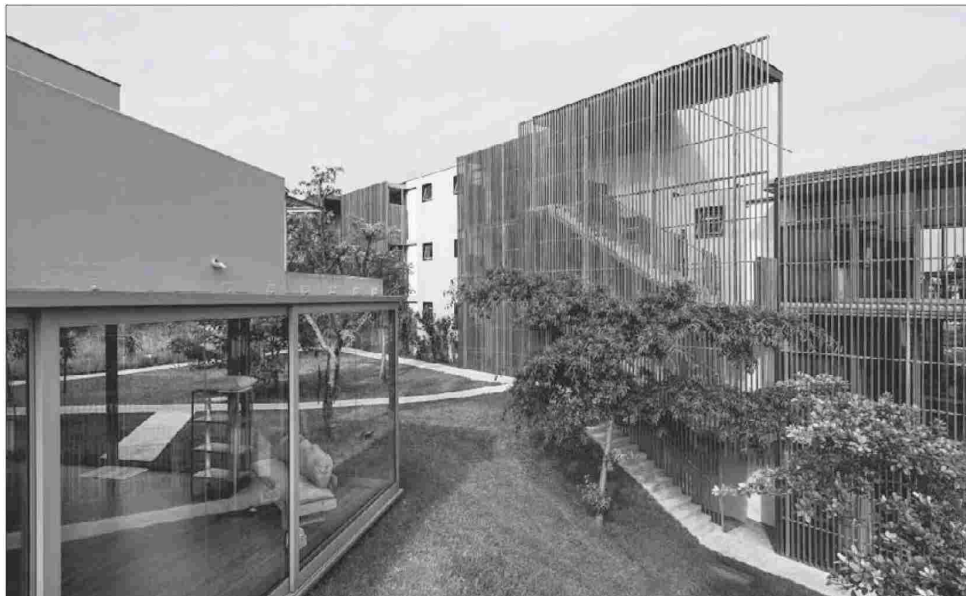
The winning design of the Dunkirk All Suites Hotel in Salt Rock.
